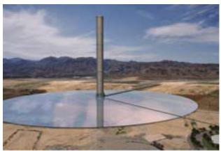
The canopy at the bottom of the tower acts like a car's windshield. Sunlight passes through it, but the heat that is generated by the ground below cannot. As a result, the air below the canopy absorbs the heat and becomes warmer.
